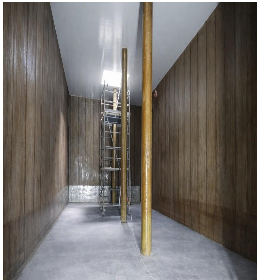
● Irrigation Tank GRP Lining
